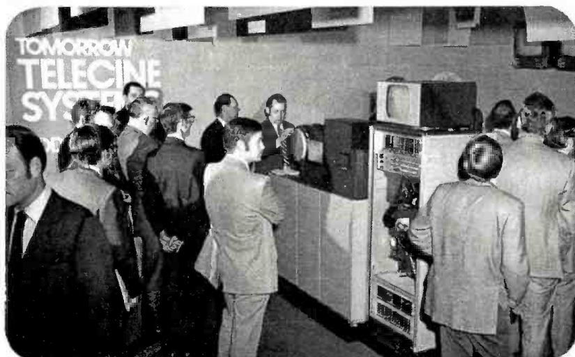
On display was a unique multiplex system with one TK-28 installed internally and the other, externally—providing a two-output color system in the same floor space normally required for a single output system.
